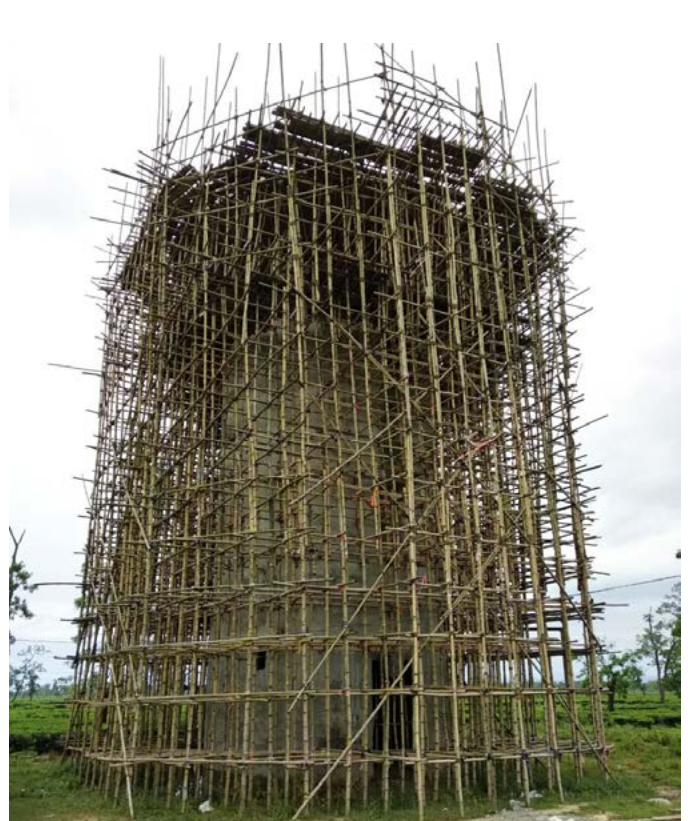
Construction of ESR in Jorhat
