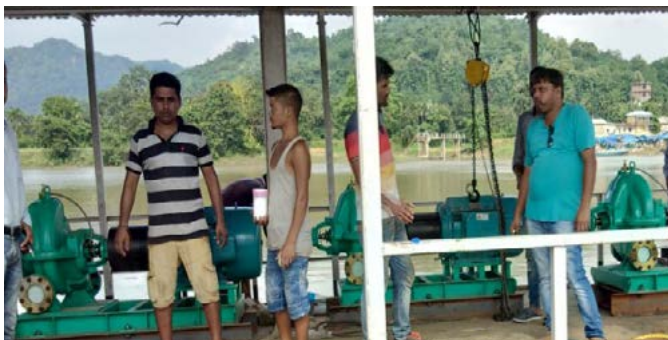
Installation of Raw Water Pump for Chandrapur WTP, Kamrup
