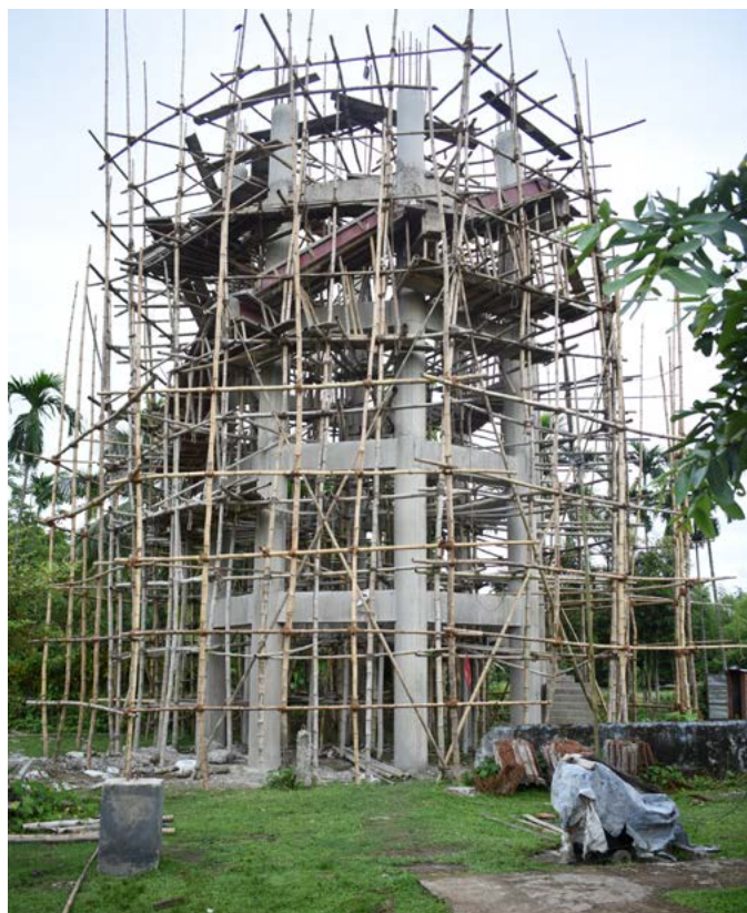
Construction of ESR in Hailakandi
