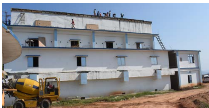
Water Treatment Plant in Dimoria, Kamrup
