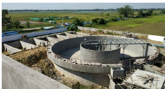
Construction of ESR in Jorhat
