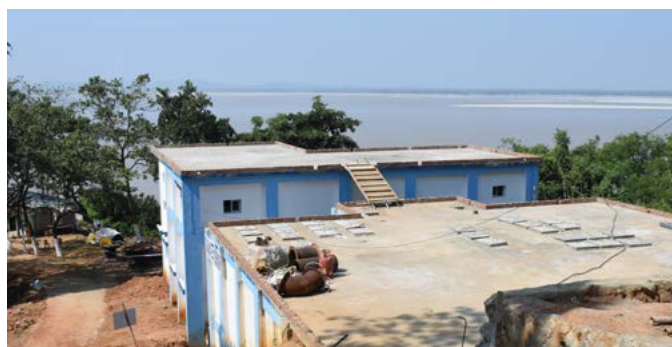
Water Treatment Plant in Chandrapur, Kamrup
