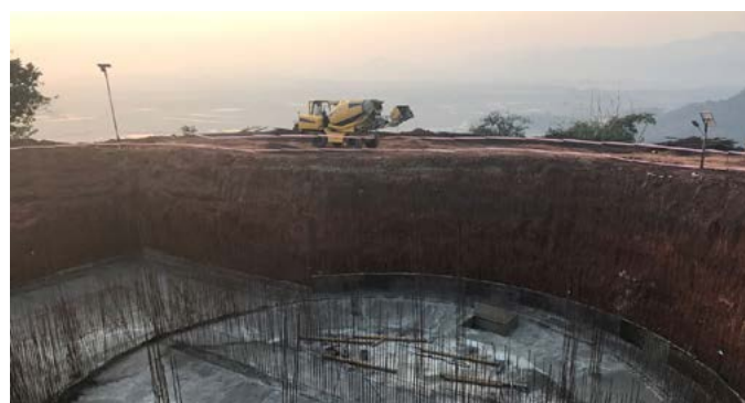
Water Treatment Plant in Dimoria, Kamrup
