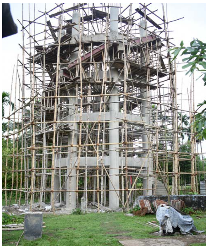
ESR Construction in Hailakandi
