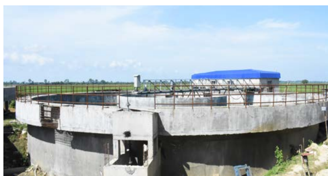
Water Treatment Plant in Jorhat
