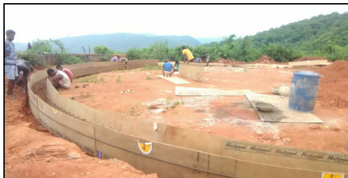
Construction of GSR in Kamrup(M)
