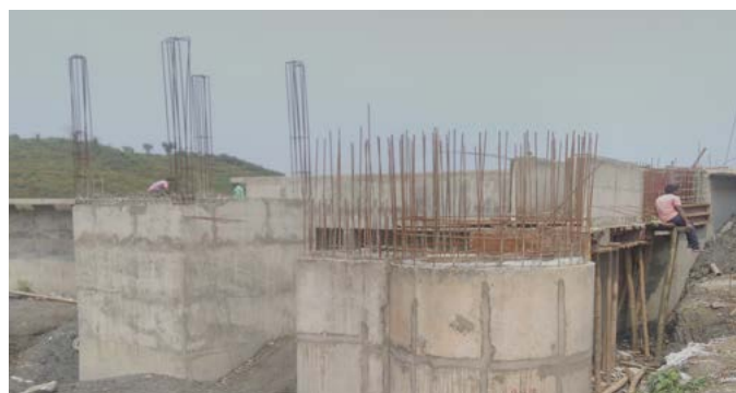
Water Treatment Plant in Hailakandi
